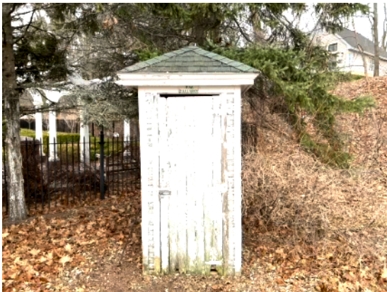
The telegraph shack before and after restoration
