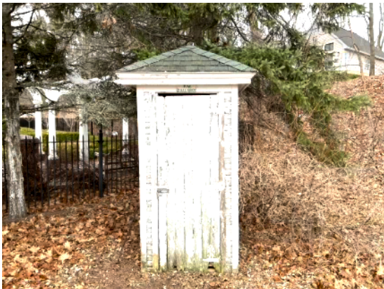
The telegraph shack before and after restoration
